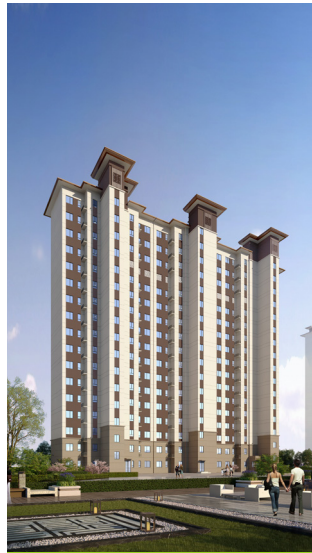
Yuejiangshan Passive Buildings Project in Xingtai, Hebei
