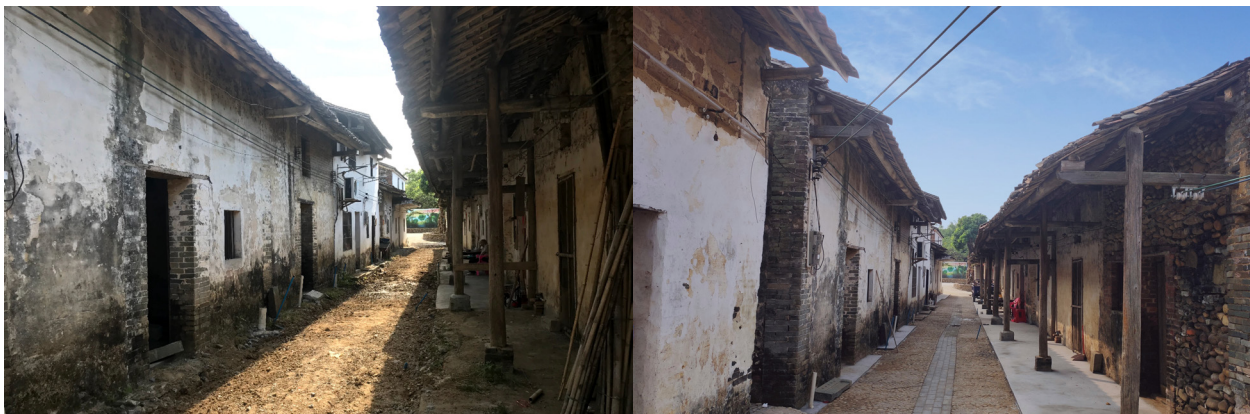
Village lanes before and after renovation in Yuzui Village, Qingyuan
