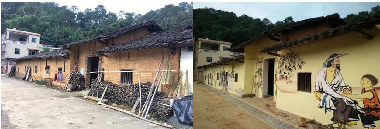
Housing appearance before and after the renovation in Lianzhang Village, Qingyuan
