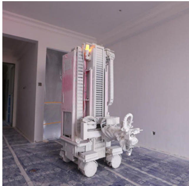
Country Garden's indoor spraying robot in operation
